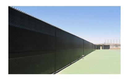
> Fabrication: 4 ply, reinforced hems on all sides with #2 brass grommets placed at 18" intervals.
